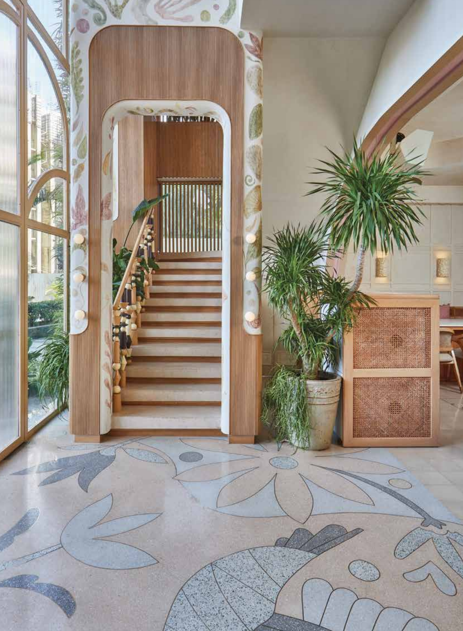
The restaurant entrance lobby flooring boasts intricate depictions of birds and flowers, beautifully outlined with a brass strips and then encased in BFT In-Situ Terrazzo. Interiors - Ruchika Chhabria
