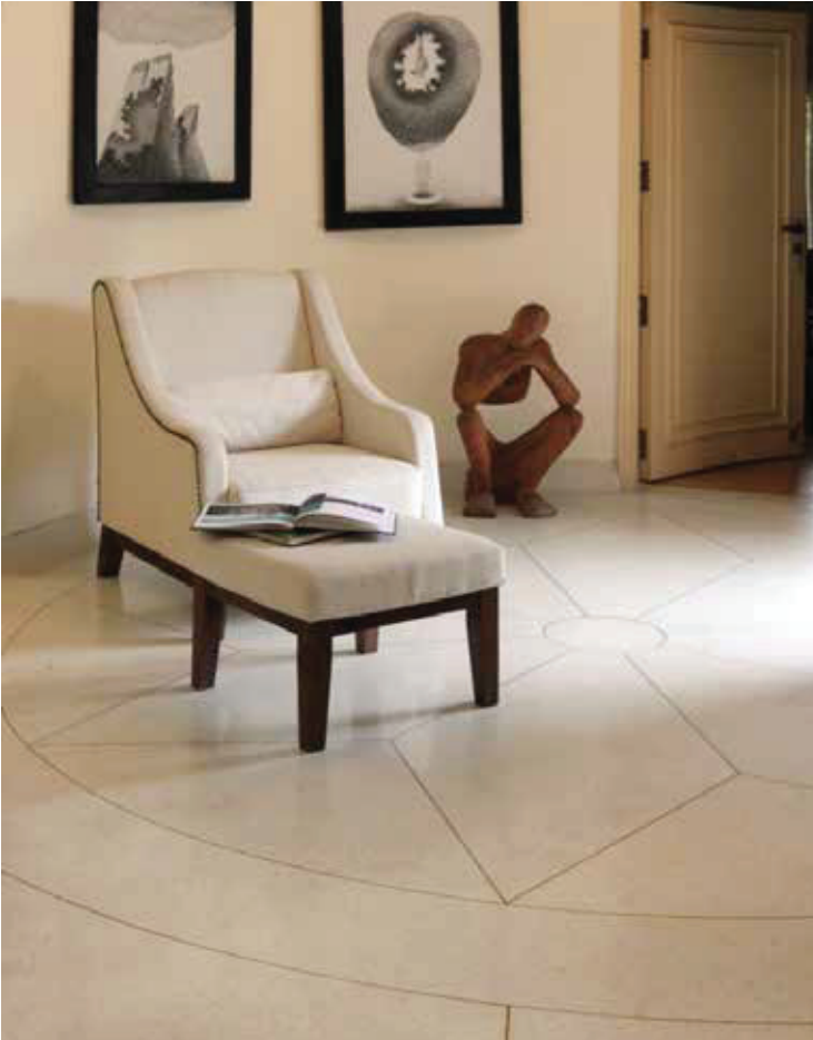
Cast In-situ Terrazzo with brass strips at this farmhouse in Delhi. Interiors - Sense by Akshi
